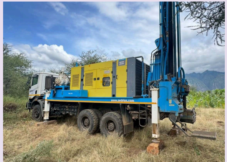
Well being drilled by WaterPro
