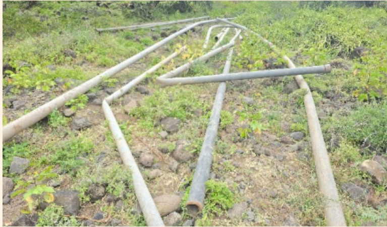
Mangled steel pipeline
