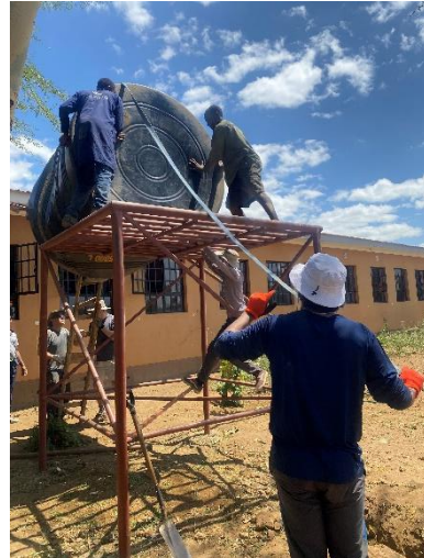
Figure 13 Lifting a water tank that is used to irrigate the school garden
