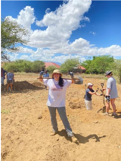
Figure 14 Digging hole 2ft within the school orchard
