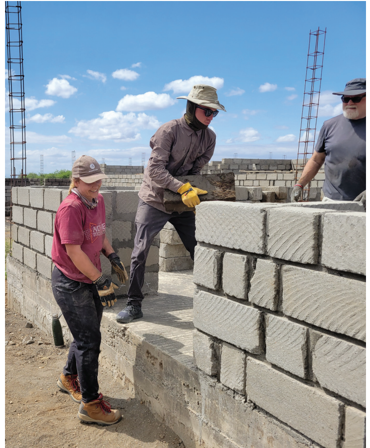
Positioning stone blocks for masons
